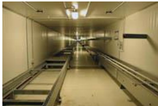
Tunnel to Distribution Facility
